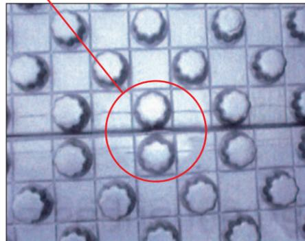
It is not required, but a good idea, to walk along the interlock area of the panels (after each couple of rows) to ensure that the panels are locked together.
