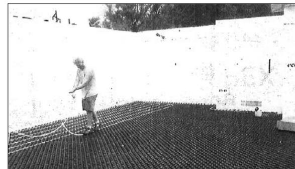
The only tip about making the PEX installation easier is that when making a turn, ensure the PEX is fully seated in the knobs before beginning or continuing a run. Other than this tip, installation is as simple as walking the tube in place.
