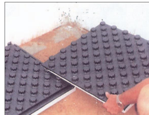
Continue placing trimmed panels until you get to the north wall. You will most likely need to cut the final panel in this row to fit into place.
