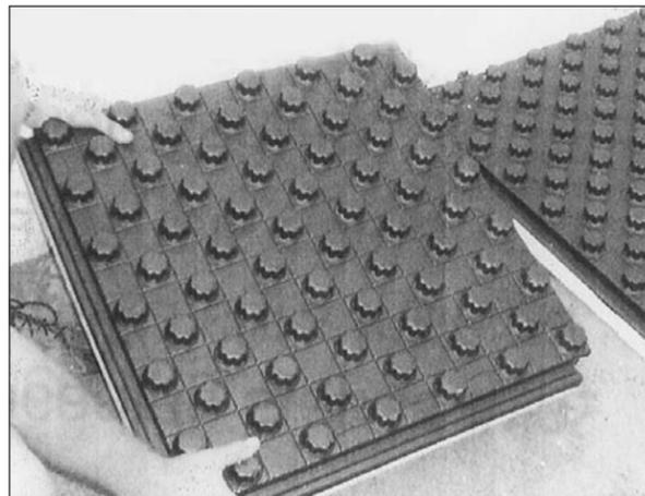
If the flat-knob-flat sequence is interrupted when beginning a new row, simply cut two more inches of the panel off. This will get the sequence back in proper order.
